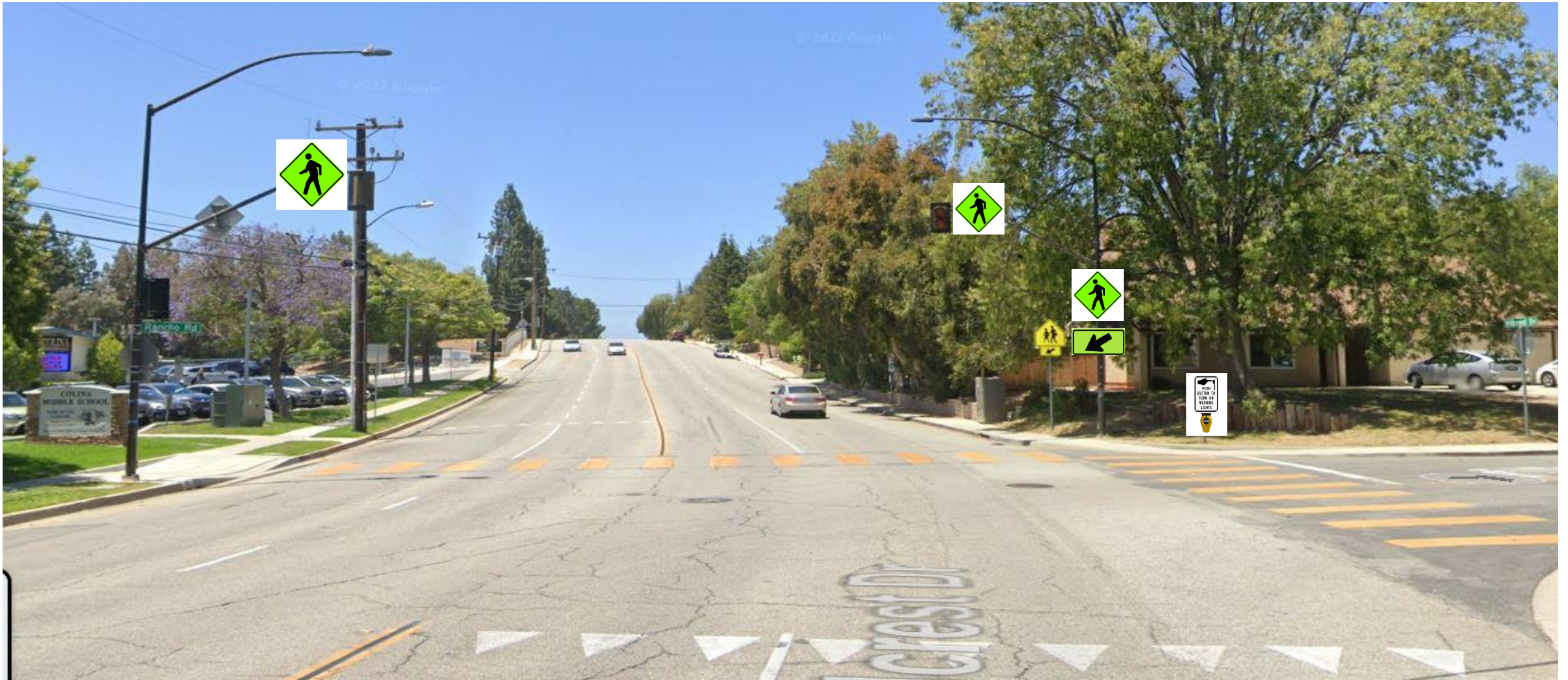
HILLCREST DRIVE - COLINA ELEMENTARY SCHOOL UPGRADES (COMPLETED FALL 2023)
